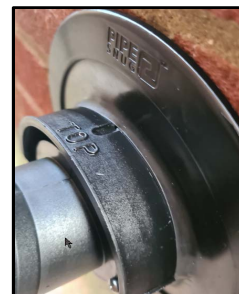
Fig 4: Shows the FlueSnug correctly located on the flue terminal.
