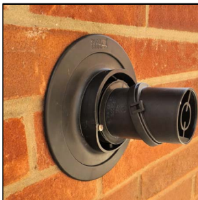
Fig 2: Shows Fluesnug installed with a Condensfit II flue.
